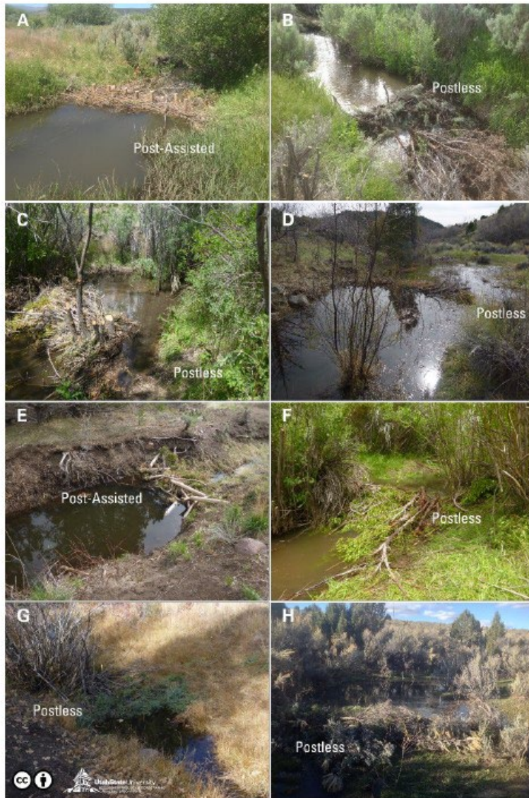
Figure 6 - Representative photos of the diversity of possible BDA shapes, sizes, locations, and building material. (A) post-assisted and willow weave (B) postless, sage and juniper (C) postless willow, using existing willow for stability (D) postless, juniper (E) post-assisted and juniper (F) postless willow and juniper (G) postless juniper (H) postless sage.
