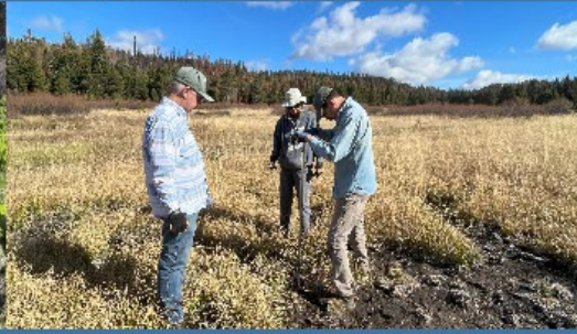
Volunteers installing groundwater monitoring wells.
