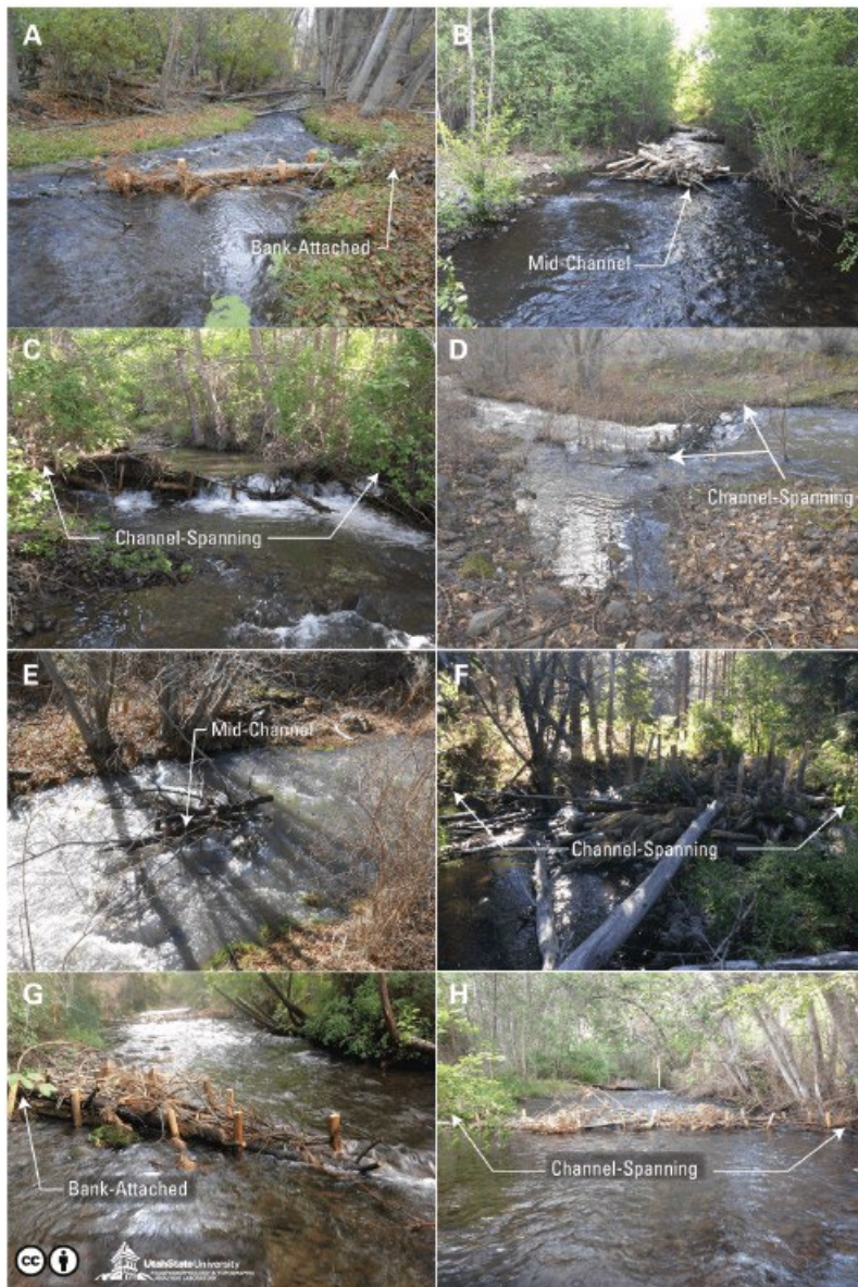
Figure 5 - PALS can be built in a range of shapes, sizes and in different channel locations. (A) bank-attached, (B) mid-channel, (C) channel-spanning, (D) channel-spanning, (E) mid-channel, (F) channel-spanning, (G) bank-attached, and (H) channel-spanning
