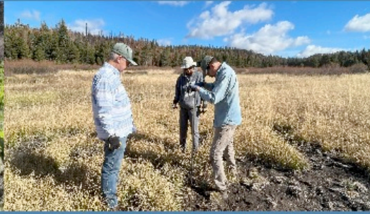
Volunteers installing groundwater monitoring wells.
